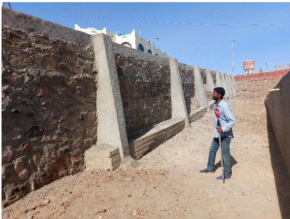
Fig 46: Area 2: Overview of the reinforced southern perimeter wall from the east.
